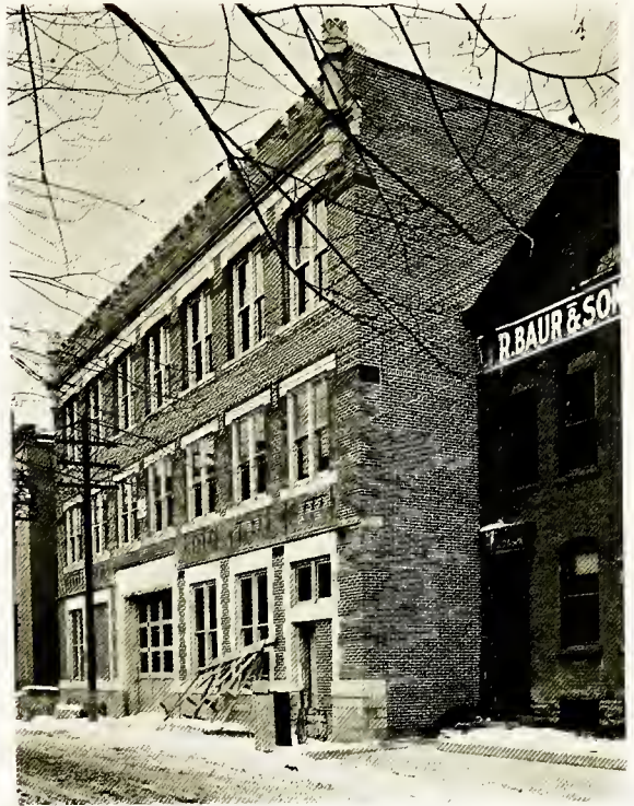
City Police Station, North State Street (Under Construction)
